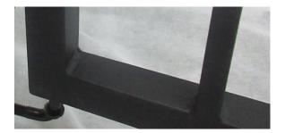
2. Attach a hinge to the bottom of the right side of the arch and the right gate – ensuring there is a nut and a washer on either side of the arch frame. Do not tight at this stage. Only put on 'finger tight' to allow for adjustment. The threaded side goes through the arch frame from inside to outer, pointing up into the gate.
