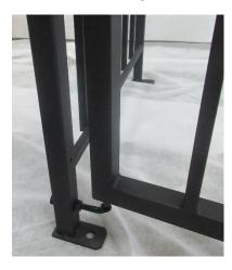
4. Attach the top left hinge in the same way as with the bottom hinges, but this time pointing down into the gate.
