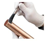
**2.** Insert the tube into the fitting until it reaches the tube stop, then wipe off any excess flux. Heat the assembled joint evenly on all sides.
