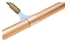
**3.** Apply solder to the mouth of the fitting. When the correct temperature has been reached the solder will flow freely and be drawn into the joint. Briefly reapply the blowtorch and wipe off any excess solder.
