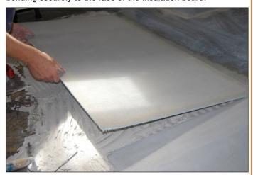
Any slight depressions or gaps in the concrete floor can normally be taken up within the thickness of the tile adhesive. Thermal insulation boards must not bridge movement joints within the sub floor. Any movement joints must be maintained throughout the construction including the boards and final floor covering. Maintain and seal all movement joints appropriately.
