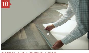
FIRST PLANKS A, THEN PLANKS B Continue each next row by placing all the planks A in a row first, followed by all the planks B. Continue in this way up to the opposite wall is reached. Fill the remaining openings as in figure 9.
