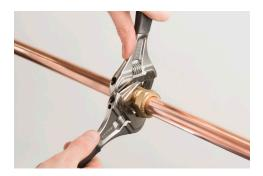
Tighten the nut further using open ended or adjustable spanners, using the spanner flats incorporated into the fitting body and nut. The second spanner must be used to prevent the fitting rotating as the nut is tightened.
