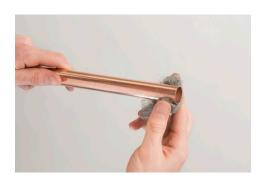
Clean the outside of the pipe, making sure that there is no pipe residue, dirt or grit is present near the joint.
