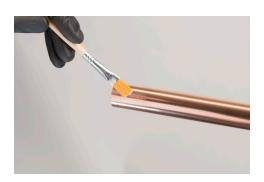
As soon as possible after cleaning, flux should be applied sparingly to the inside of the fitting and also the outside of the pipe at the point of overlap. This will help the capillary action and induce a stronger joint.
