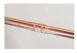
Insert the tube into the fitting until the pipe reaches the base of the pipe stop. A small twist can also be applied to ensure even coverage of the flux. At this point, excess flux should be wiped away using a rag.
