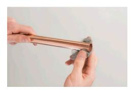
Clean the outside of the pipe, making sure that there is no pipe residue, dirt or grit is present near the joint. Failure to remove all oxides and any material where the fittings and tube overlap can interfere with the capillary action and thus will reduce the strength of the soldered joint, resulting in failure.
