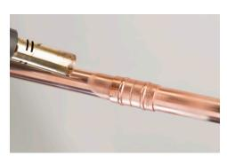
When heating, the entire circumference of the fitting should be heated evenly. It is recommended that you preheat the pipe and the fitting before applying direct heat.
